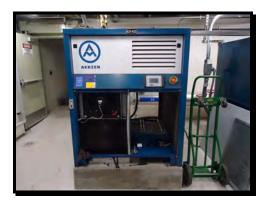
• Rebuilt both ammonia feed injectors.
